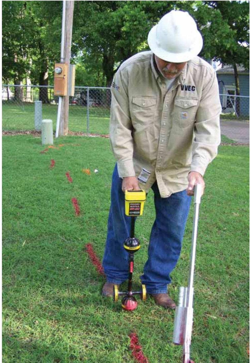
*VVEC Serviceman Mike Dickey marks a member's underground electric lines with red paint so the member's in-ground swimming pool can be installed without cutting the line and interrupting electric service. Members can dig up to two feet on either side of the red line.*
