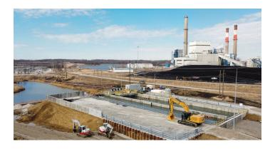
This concrete tank allows fly ash to be recycled and water reused at the Thomas Hill Energy Center. Photos courtesy of AFCI
