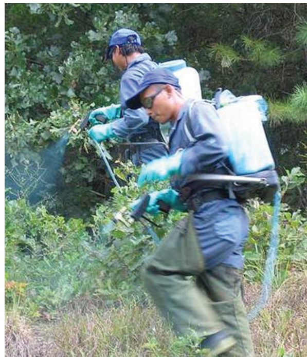
Contractors carry four-gallon backpacks (above) and use wands to apply the herbicide where it needs to go to treat growth and vegetation growing in the co-op's right-of-way. Areas served by the Ramona, Vera, Oologah, Green and Watova substations (below) are targeted for the herbicide-spraying program this summer.
